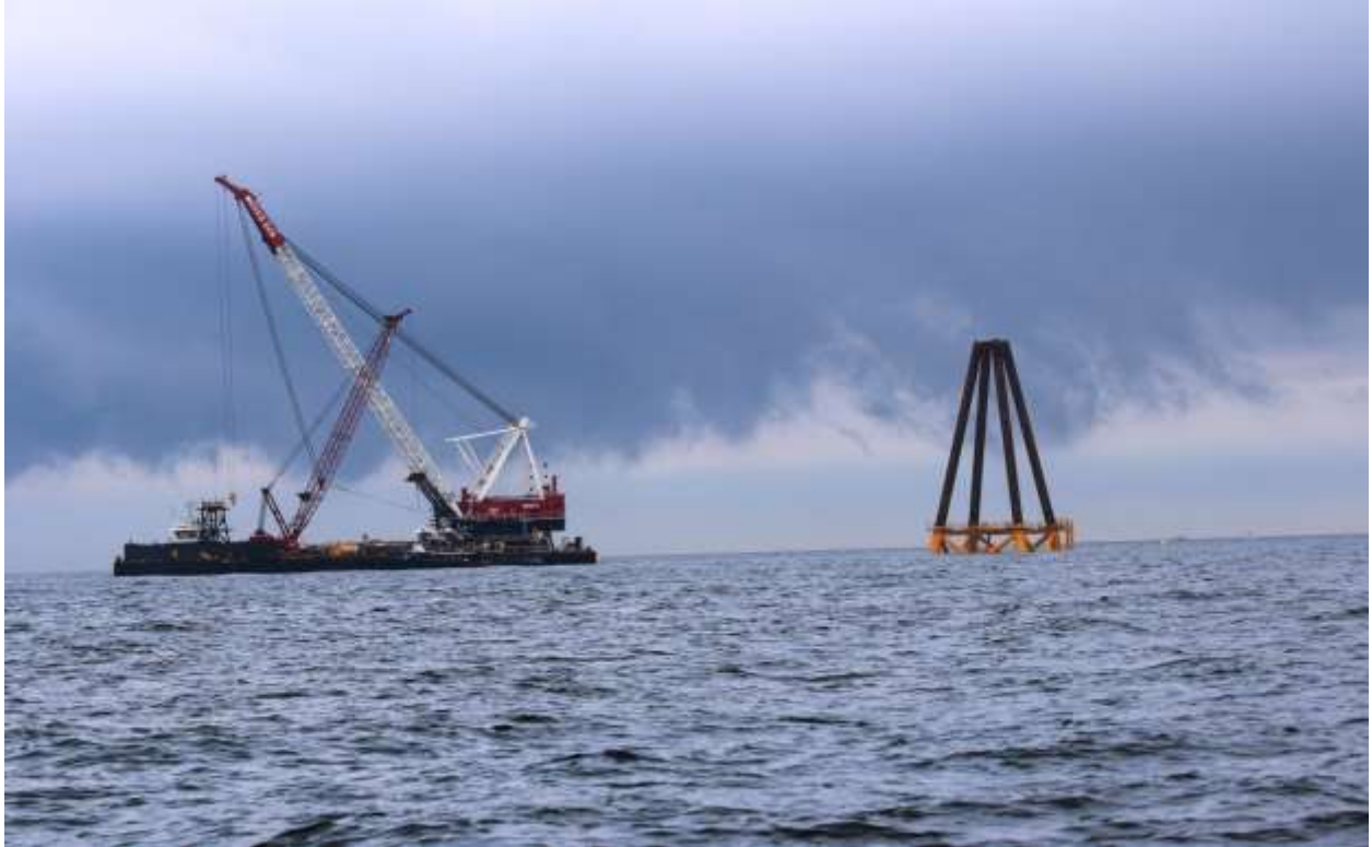
Figure B-21.9/20/2015 Offshore Photo 2579: Weeks Barge 526 next to WTG 5 with second set of piles in place.
