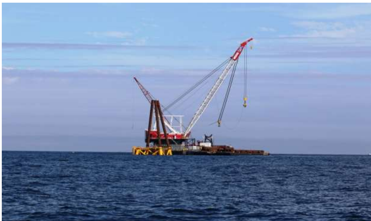
Figure B-10. 8/23/2015 Offshore Photo 0186: Weeks Barge 533 just placed third pile at WTG 3.
