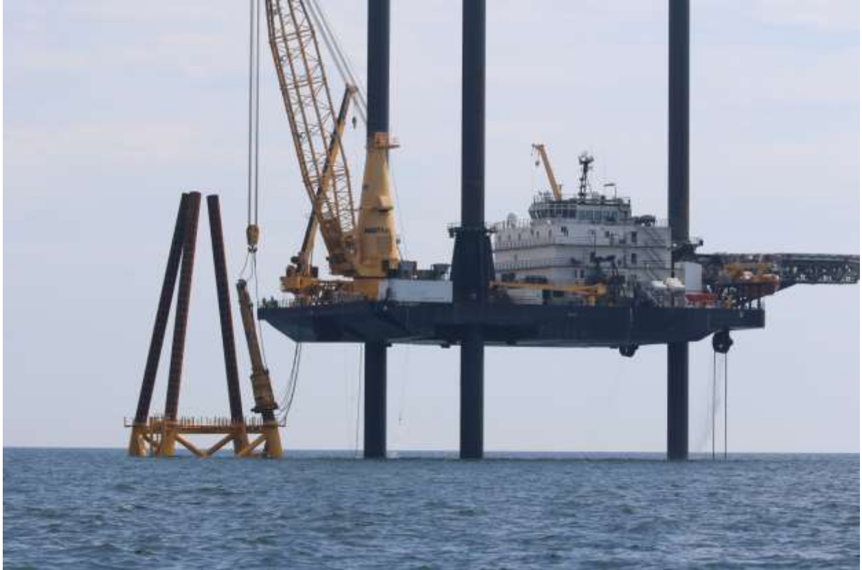
Figure B-17.9/17/2017 Offshore Photo 2352: Lift Boat Roberts driving the first pile at WTG 5.
