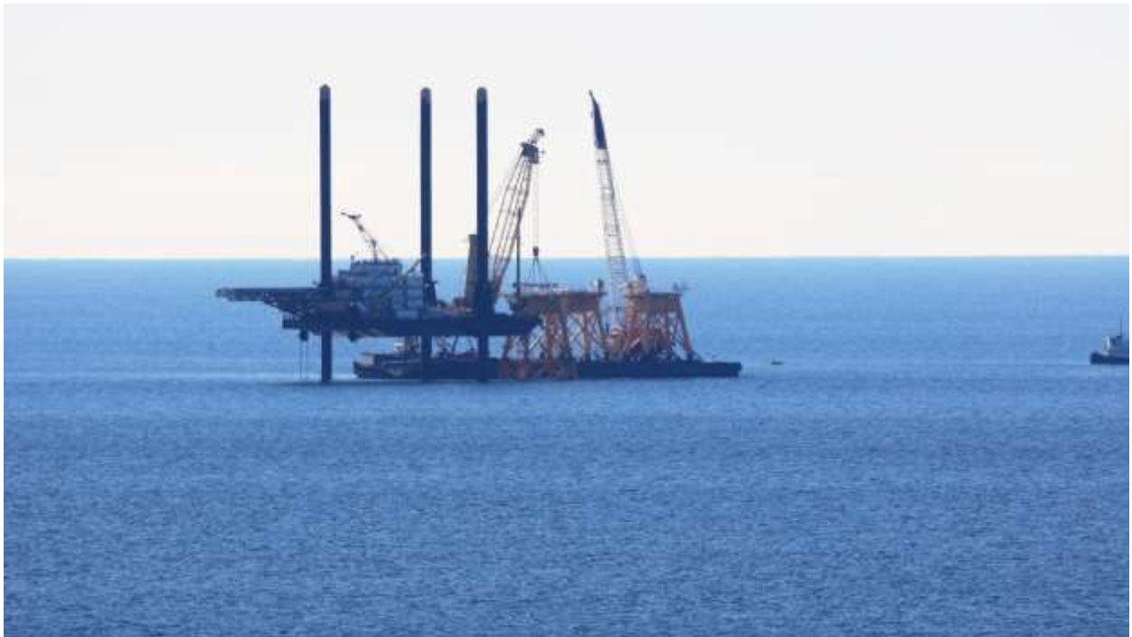
Figure B-18.11/09/2015 Onshore Southeast Lighthouse Photo 2591: Lift Boat Roberts placing transition deck at WTG 4.
