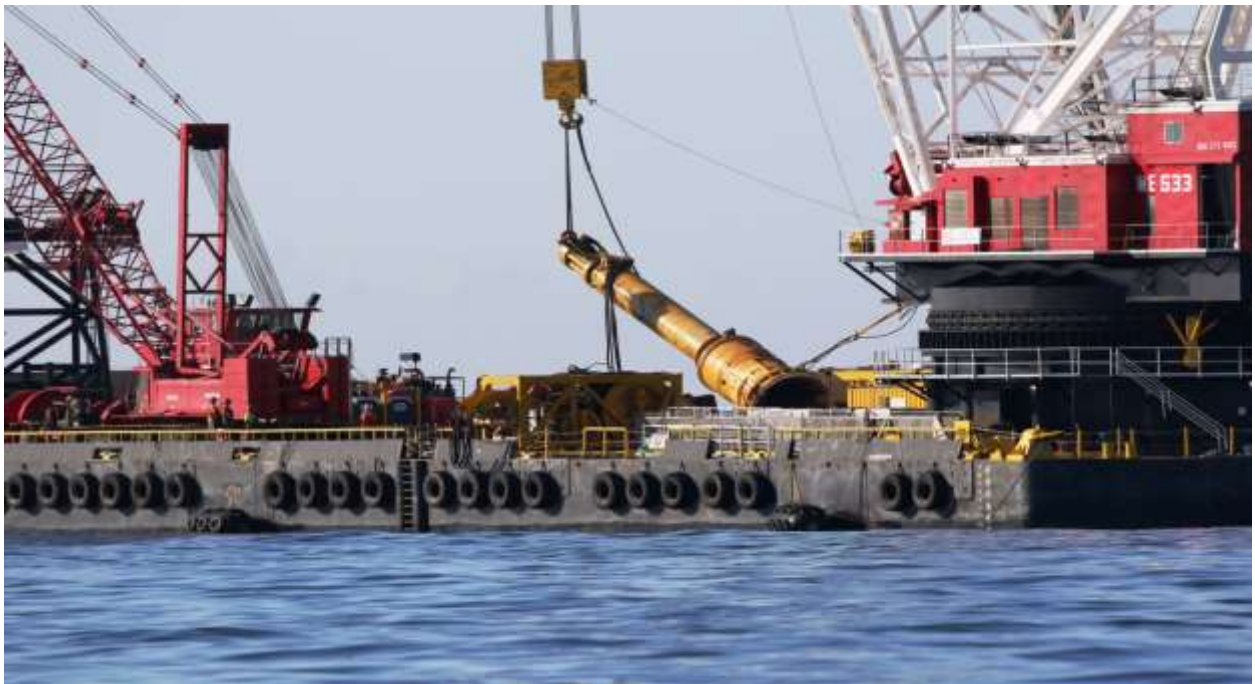
Figure B-12.8/29/2015 Offshore Photo 0622: Hydraulic hammer being lifted from Weeks Derrick Barge 533.
