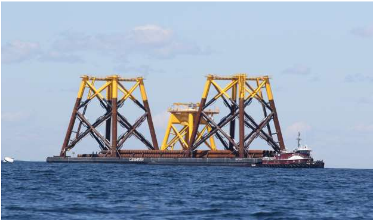
Figure B-8. 8/15/2015 Offshore Photo 0014: Two foundations, WTG 2 transition deck, and piles aboard the Cashman barge with support tug Reed Danos. Anchor buoy visible.
