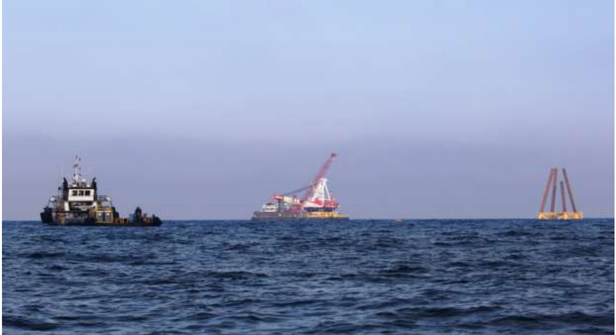
Figure B-11.8/26/2015 Offshore Photo 0581: Supply vessel Josephine Miller and Weeks derrick barge 526 at WTG 2. WTG 3 is to the far right with four piles ready to be driven.
