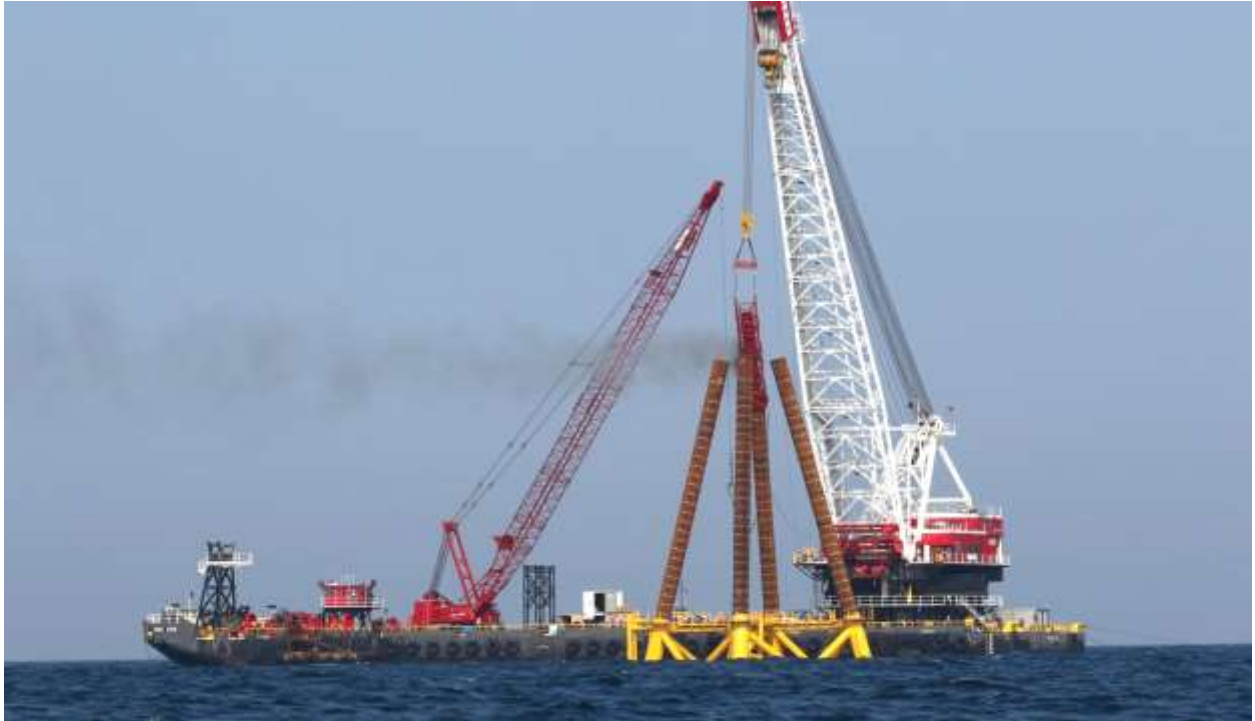
Figure B-5. 08/18/2015 Offshore Photo 0111: Weeks Barge 533 piling at WTG2 with diesel hammer (notice smoke).
