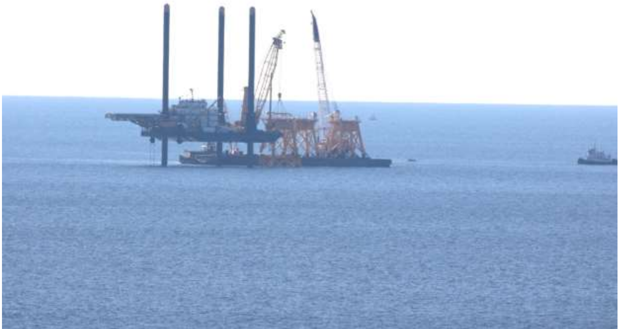
Figure 18. Transition deck installation.
