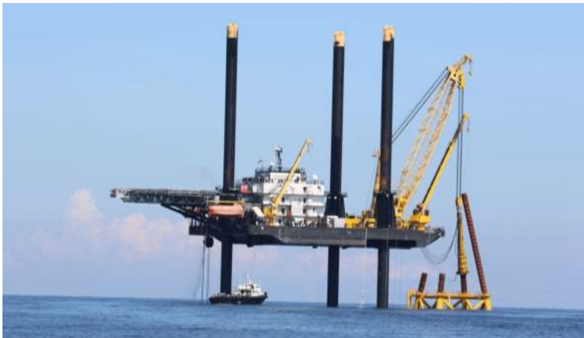
Figure 17. L/B Roberts hammering piles at WTG 1.
