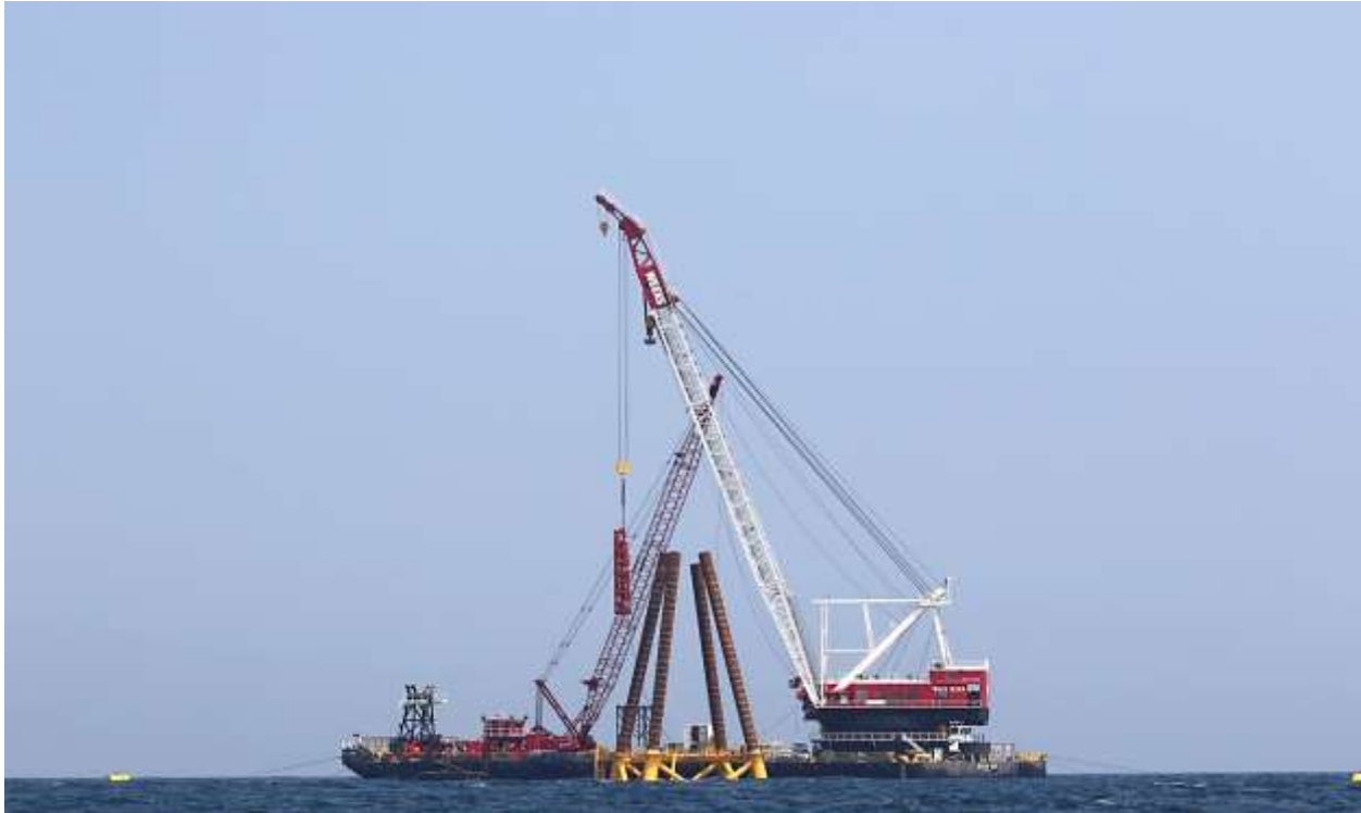
Figure B-7. 08/18/2015 Offshore Photo 0111: Weeks Barge 533 removing diesel hammer from piling at WTG2.
