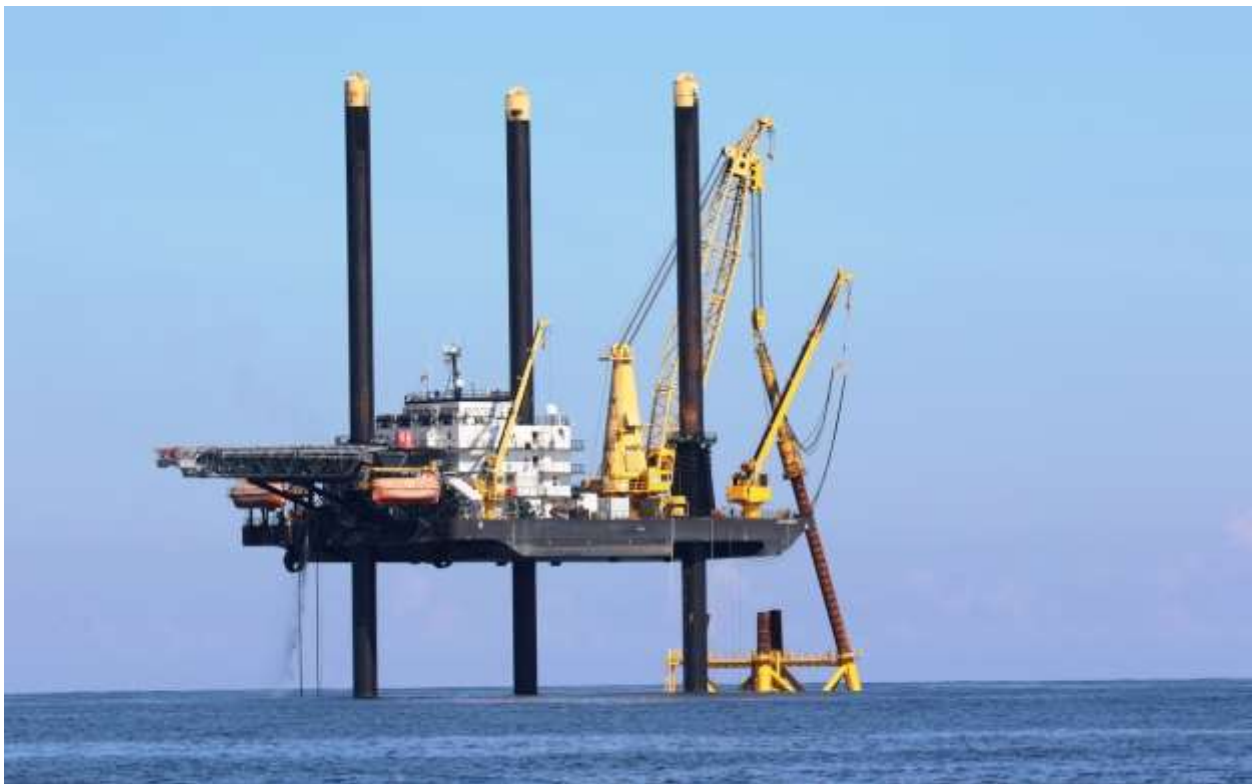
Figure B-16.9/19/2015 Offshore Photo 2542: Lift Boat Roberts driving the last pile at WTG 1.
